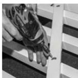
**STEP 15** - Once all of the screws have been installed into the balusters thru the cross brace, snap a plug into each hole. Apply firm pressure with your thumb and the plug should "snap" into place.
