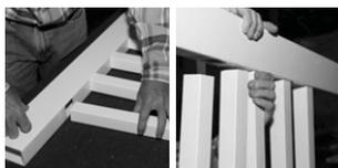
**STEP 5** - With balusters in place start with one post and slide both rails into the gate pockets, then slide the other side into the pockets. Ensure that both sides fit snugly against the back of the gate pocket and **check your finished gate width measurement.**
