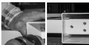
**STEP 7** - Place a square in the corner where the bottom rail meets the post. Make sure you have a 90° angle between post and bottom of rail. Alternatively use a tape measure and measure diagonally across the gate from the top of the opposing post, to the bottom of the other. Do this for both sides. They should measure the same. If they do not; you may have to tap/push one side up or down.
