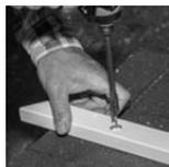
**STEP 14** - With the 5/8" drilled holes facing up install a screw through the bottom of the cross brace into the baluster. Repeat this step, for each of the three holes.
