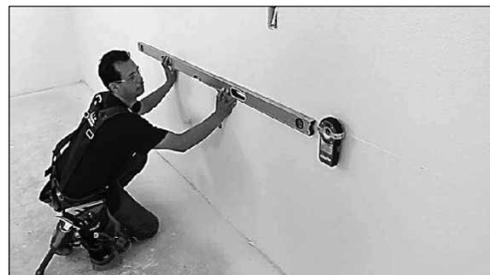
4. Find and mark the studs. This can be done by trial and error of driving a nail in the wall until you find a stud or use an electronic stud finder. Studs will usually be every 16" center to center.
